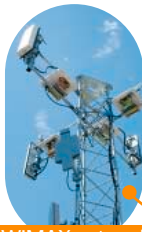
Towerstream's WiMAX network can deliver a 5- to 10-mile ring of high-speed Internet service.
