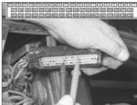
16.7a Connect the ohmmeter probes to terminals 7 and 12 (later Motronic systems) of the ECU connector and check for a smooth change in resistance as the door on the airflow meter is slowly opened and closed
