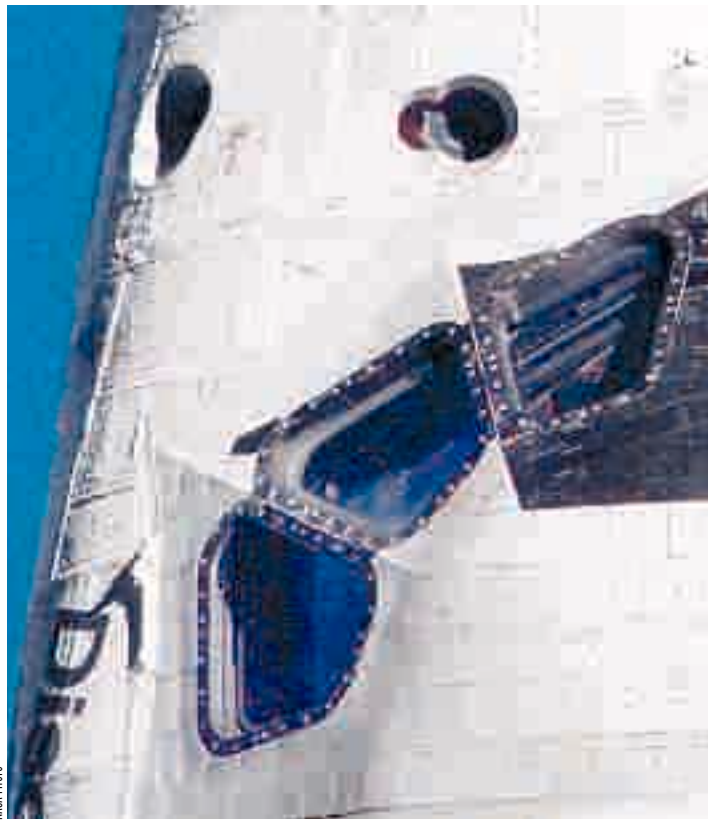
This photo of the shuttle Discovery, taken from the international space station, shows the damaged thermal blanket just above the "D" in Discovery under the orbiter's crew cabin window.
