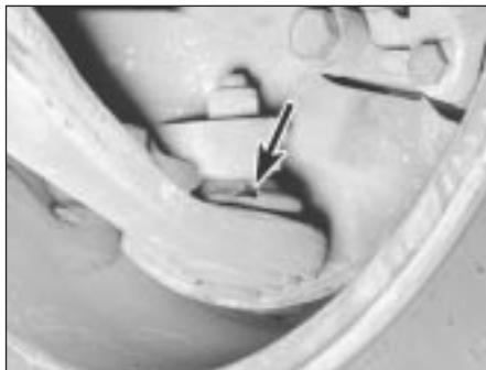
24.10 Inspect the balljoint boots for tears (arrowed)
